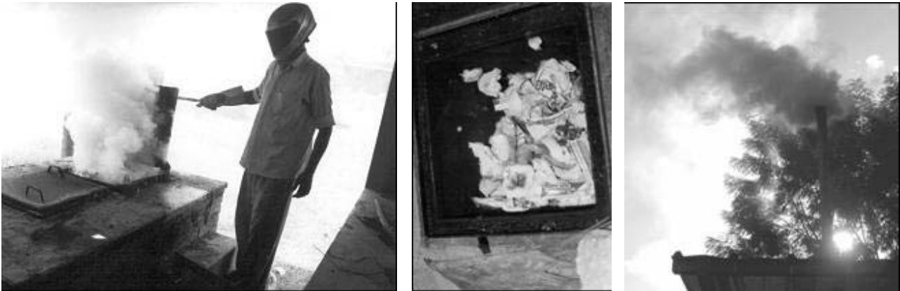
Figure 2 Photos indicating construction problems for De Montfort Incinerators in Kenya.
